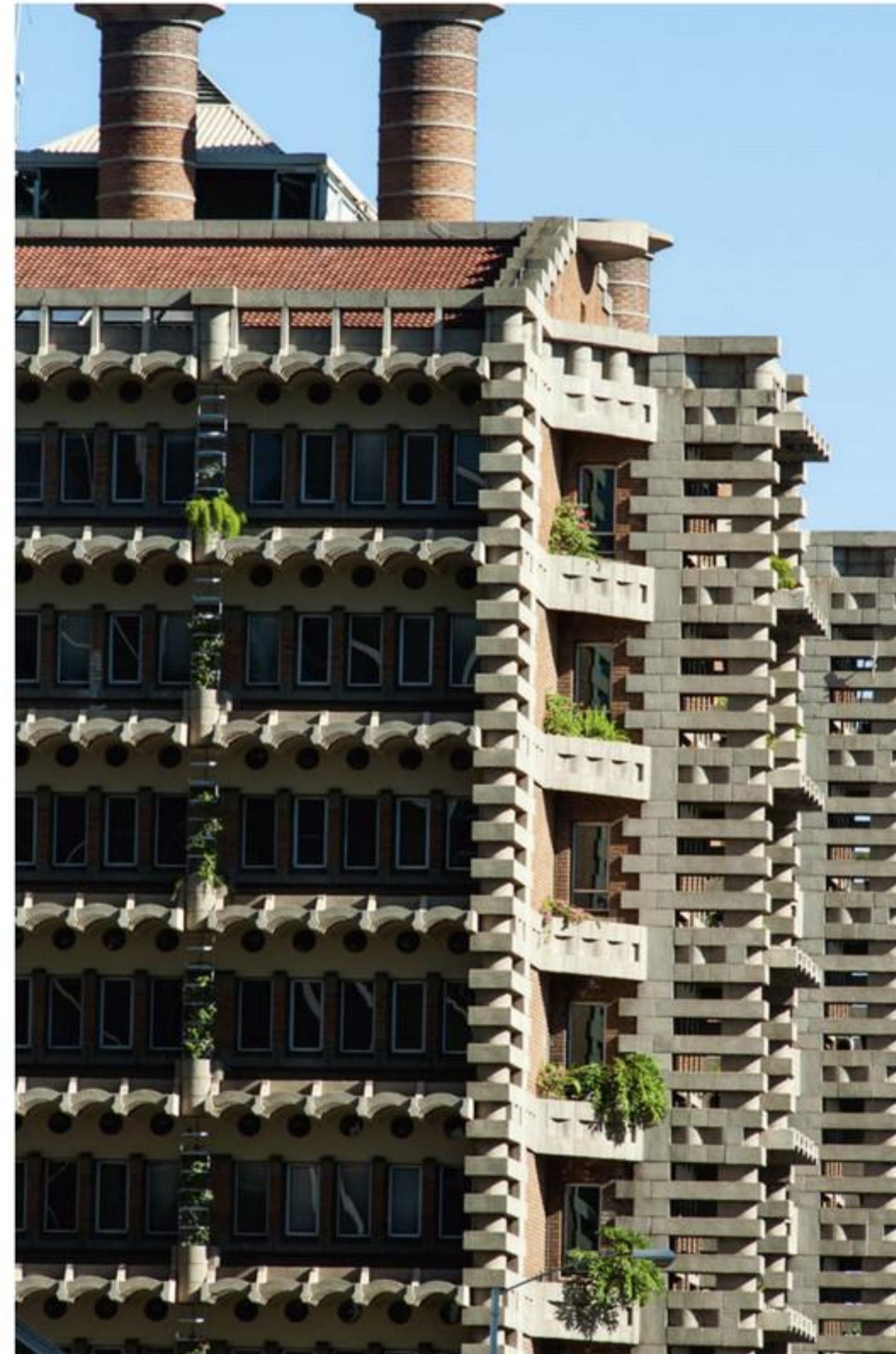
2 Eastgate Building in Harare, Zimbabwe
