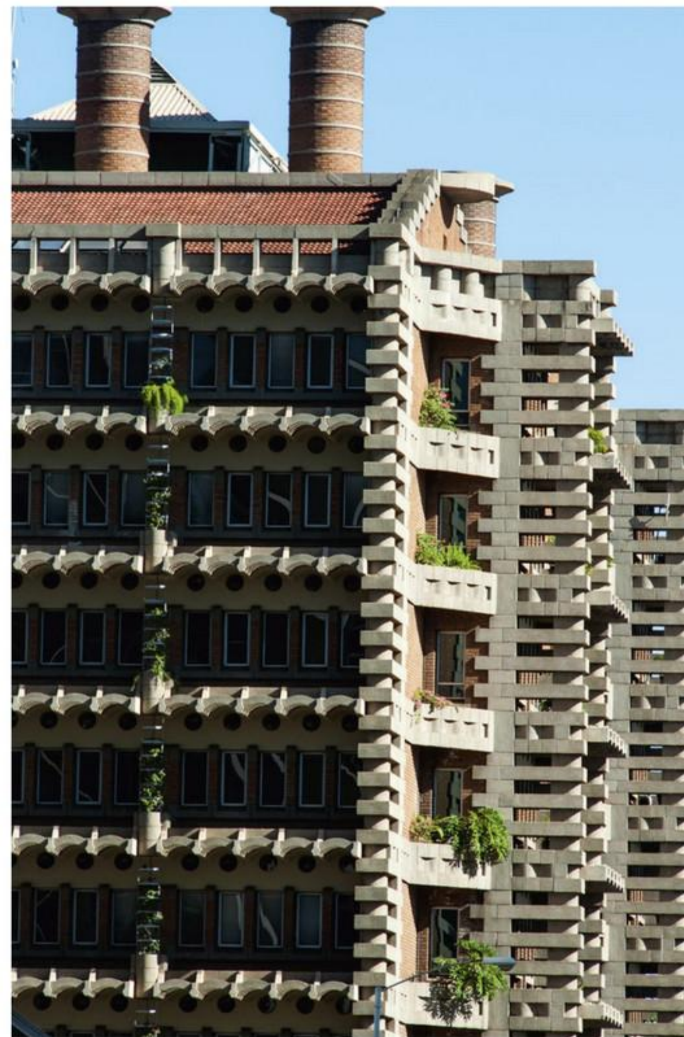
2 Eastgate Building in Harare, Zimbabwe
