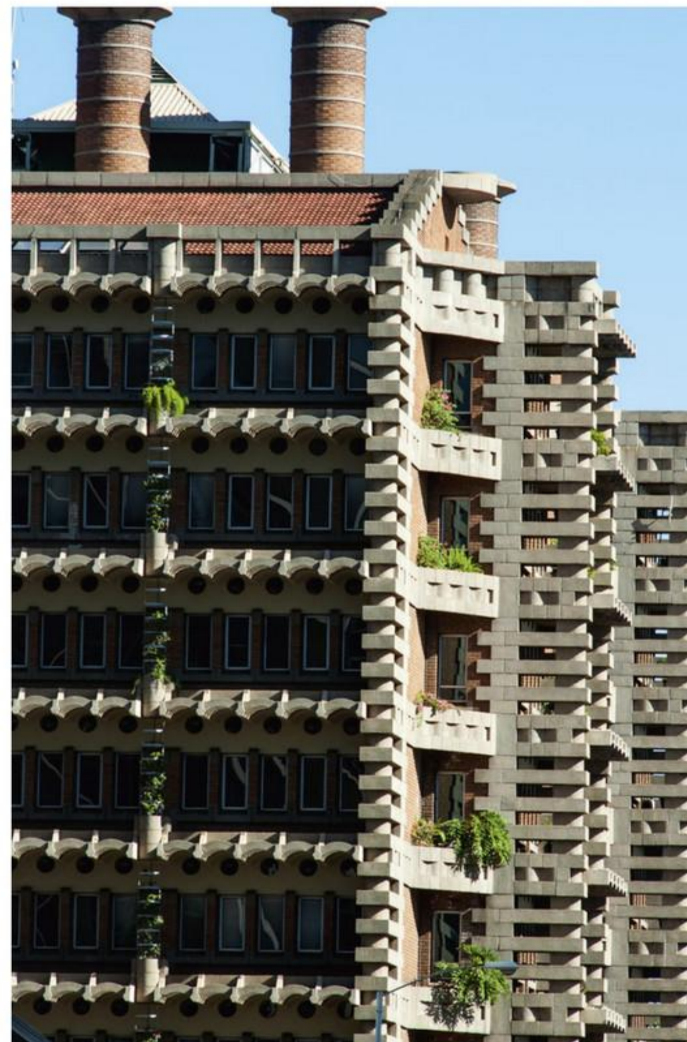
2 Eastgate Building in Harare, Zimbabwe
